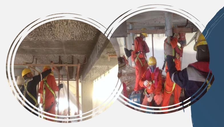
Vortex team rose to the challenge of enabling an existing jetty to withstand an operational loading arm with a significant increase of MLA size based on the original design. Our marine team had to perform the reinforcement work for critical coring, installation of studs and anchors and marine grouting under constrained conditions. The final quality reflected our team's outstanding workmanship and in-depth knowledge of such critical marine work.
