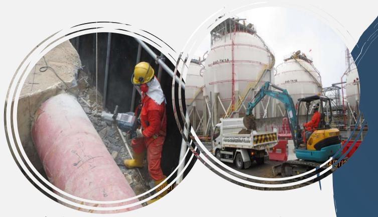
Vortex's plant maintenance team was put to a test during an actual emergency when the safety of the plant's operational readiness was compromised. During a leakage of the underground Firewater Line, our team reacted speedily by obtaining the necessary endorsements for documentation of work to be carried out in confined spaces and accurately enforcing the methodology of performing civil works without aggravating the existing damaged condition.
