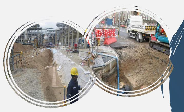
As part of the early works for the Butadiene Unit Project, our team supported the geotechnical works and ground engineering to allow our client to have a better understanding of the current ground conditions, which allows the engineering team to be able to design the foundation based upon the loading calibre. The range of work not limiting to boring, cone penetration and trail trenching works projected an influx to the manpower team.
